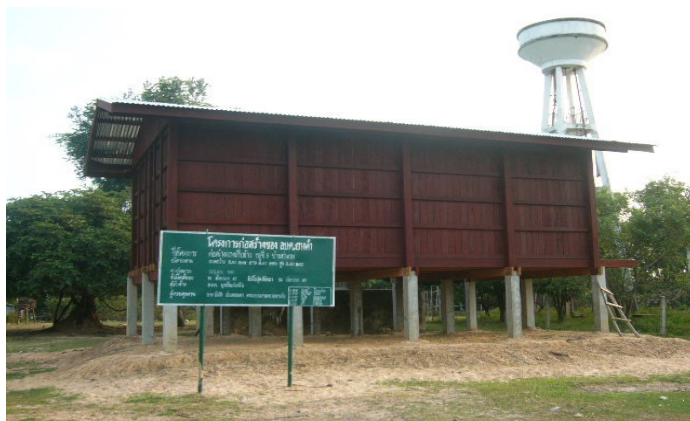
Figure 3 Water supply tank and granary of village
